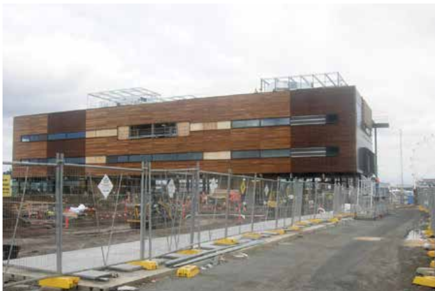
A library under construction built using CLT.
