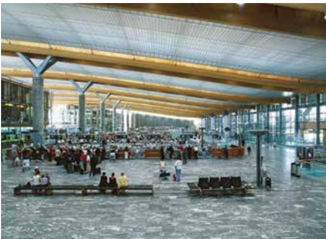
Extension of Oslo-Gardermoen Airport used glued laminated timber.
