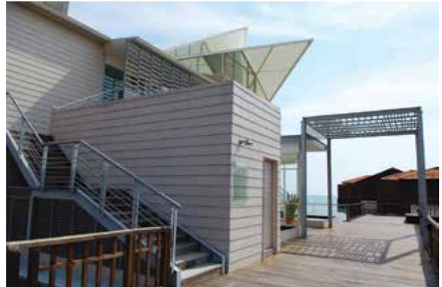
Wood buildings are easy to renovate, expand and adapt to changing uses.
