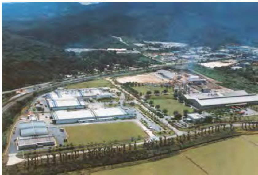
Dongwha fibreboard plant in Nilai, Negeri Sembilan.
