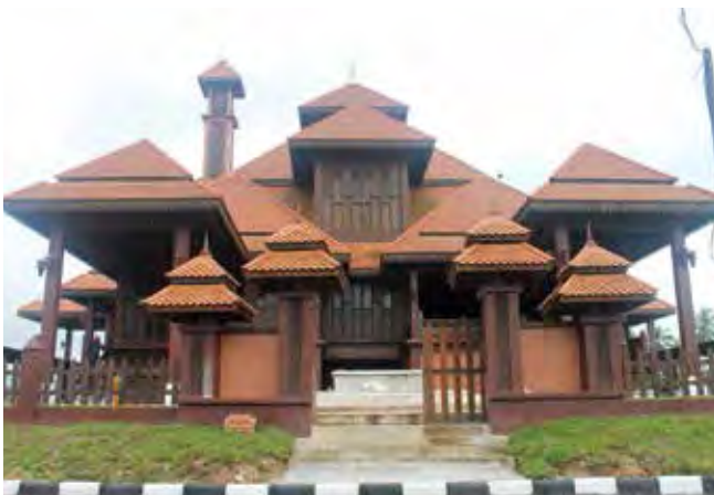
Chengal is one of the timber species being used in the Masjid Kayu, in Seberang Jertih, Terengganu.
