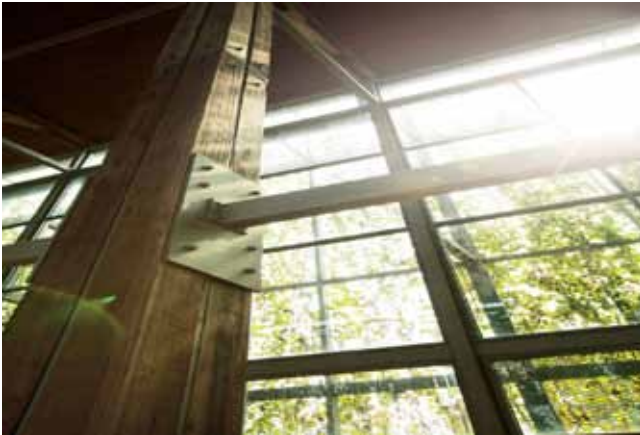
Chengal's superior strength and durability makes it useful in structural construction such as columns, beams and roof trusses.
