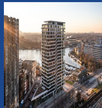
HAUT Amsterdam – The tallest hybrid building in the Netherlands
