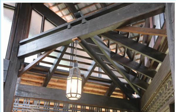
Intricate details at roof developed by the master carpenter
