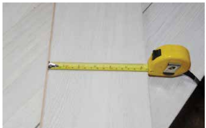
Inspection of timber size.
