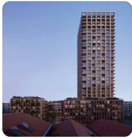
Valbella Resort in Lenzerheide, Switzerland, with modular prefabricated elements and larch wood facade
