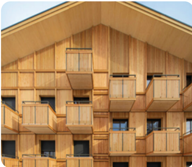
Rocket&Tigerli building in Winterthur, Switzerland, the world's tallest cross-laminated timber (CLT) building.
