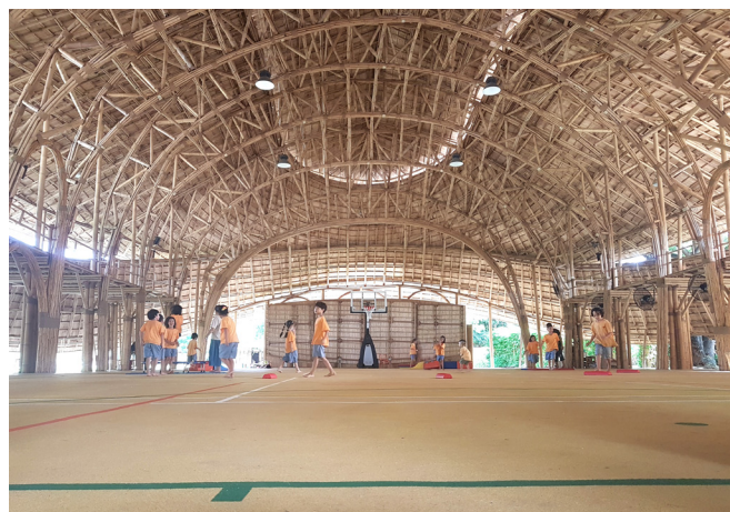
The hall of Panyaden International School using bamboo.
