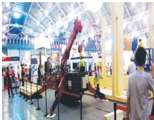
Demonstration on installation of mock up cross laminated timber using high technology machines during exhibition.
